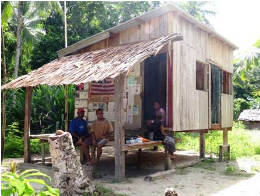
The solar panelled charge and resource centre that we built with them in 2013 was working well.
